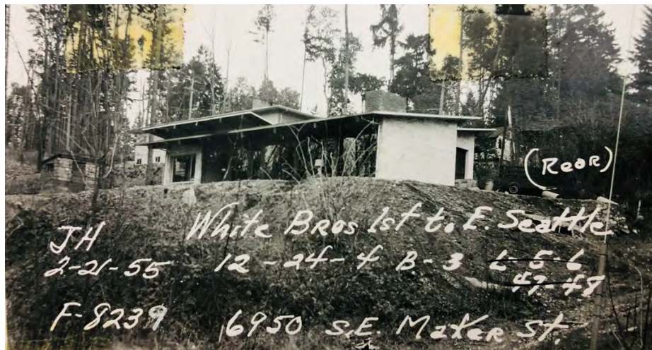
Ca. 1955 view of south (front) and west (rear yard) elevations of 6950 SE Maker Street depicting extensive fill material sloping to foreground prior to rockery placement. Note the lack of native vegetation. Present day Maker Street is in lower right of photo.
